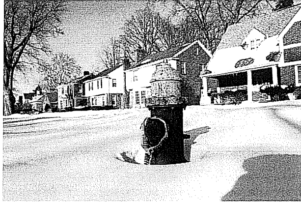
Broken hydrant in front of occupied houses at Stahelin and Eaton. Steve Neavling/MCM
